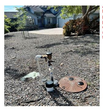
A PVB must be installed at least 12" above the highest downstream point. A PVB does not protect against back pressure. If the irrigation piping is higher downstream, the elevation causes back pressure. This PVB is installed at the highest point on the property achieving the minimum 12 inch elevation difference.
