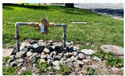
This RP is on a dedicated irrigation service line. It is installed immediately following the meter minimizing the risk of inadvertent taps into the line prior to the backflow prevention assembly. There are shut off valves and unions before and after the assembly to facilitate winterizing and replacement in the future.
