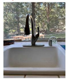
Every sink faucet is (or should be) mounted so the water enters the sink above the fill line of the sink with a separation of at least two pipe diameters. Fill spouts for swimming pools, spas and decorative ponds have (or should have) air gaps.
