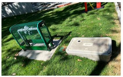
This example of installation of an RP for meter protection on an irrigation line. While it may not be at risk of freezing, the brass in backflow preventers have been a target for thieves. Consequently, it is good practice to provide locked enclosure covering assemblies.
