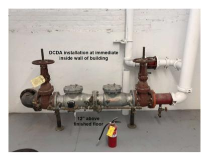
This double check backflow assembly equipped with a bypass arrangement containing a smaller double check backflow assembly, and water meter. Fire systems are not usually metered as they typically only have flow when it is activated or being tested, the detector assembly monitors for low flows. This assists in determining if there have been leaks or taps downstream of the assembly.
