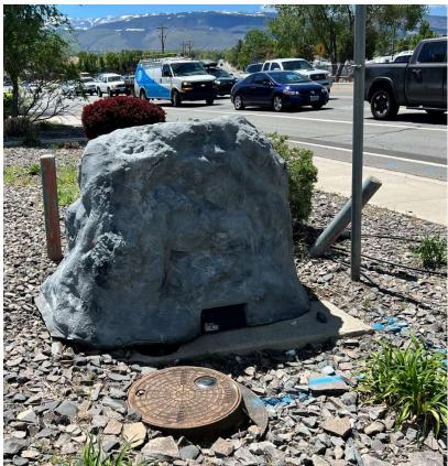
This service line to a business has an RP installed immediately following the meter. However, because of the freezing winter temperatures, this device is covered with this "fake rock", a commercially available enclosure, to protect and insulate the assembly. Note the opening at the base is intended to allow for discharges from the RPA relief port to flow out.
