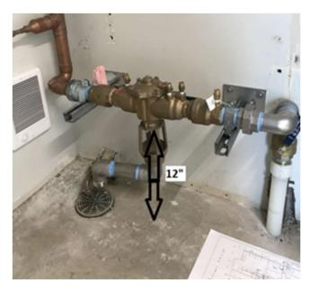
This RP was installed as retrofit application inside a building at the water riser just as it comes into the building. There are no connections allowed upstream of this assembly. The assembly is 12 inches from the wall and 12 inches above the finished floor. It is positioned such that it can be easily tested and no part of the assembly will be submerged.
