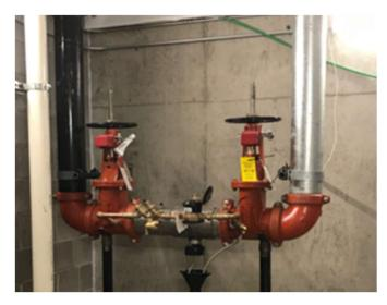
This reduced pressure backflow assembly equipped with a bypass arrangement containing a smaller reduced pressure backflow assembly, and water meter. Fire systems are not usually metered as they typically only have flow when it is activated or being tested, the detector assembly monitors for low flows. This assists in determining if there have been leaks or taps downstream of the assembly.
