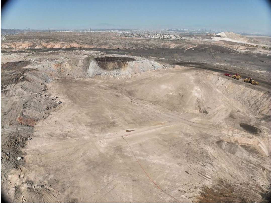
Tailings Pond 3 West – July 25, 2024
