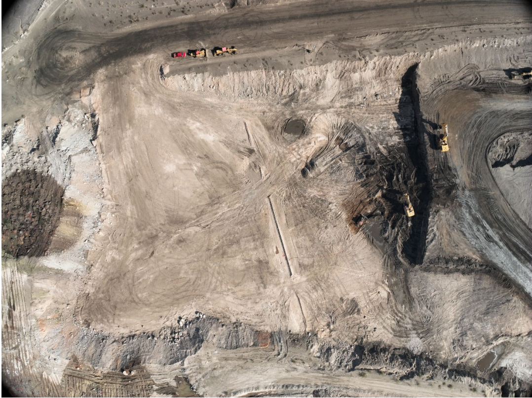
Tailings Pond 3 West – July 25, 2024
