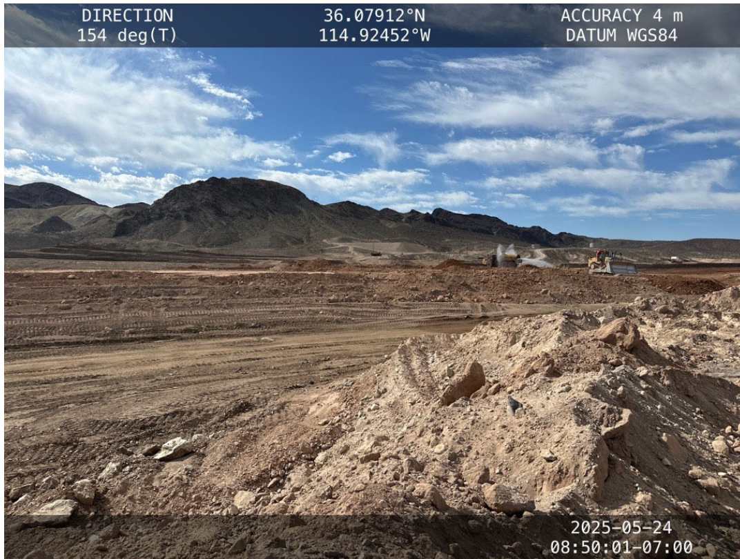
Cover Placement in Closure Unit 1 – May 24, 2025
