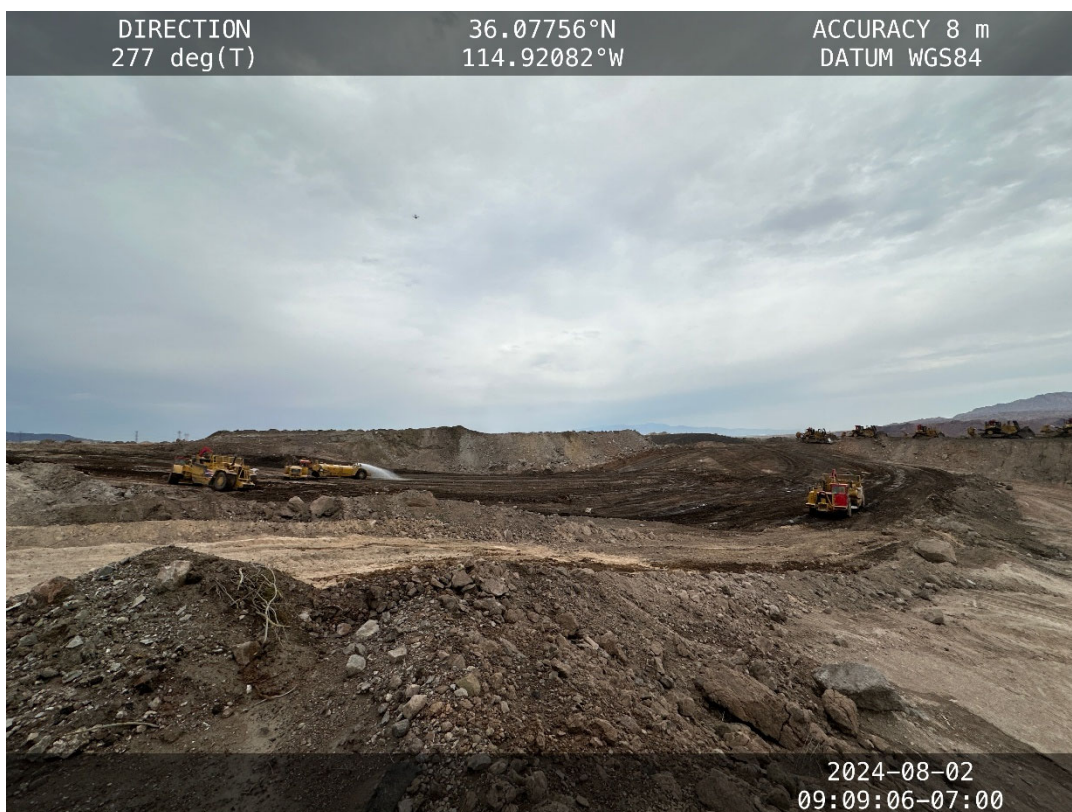
Waste Rock Reclamation in Tailings Pond 3 West – August 2, 2024
