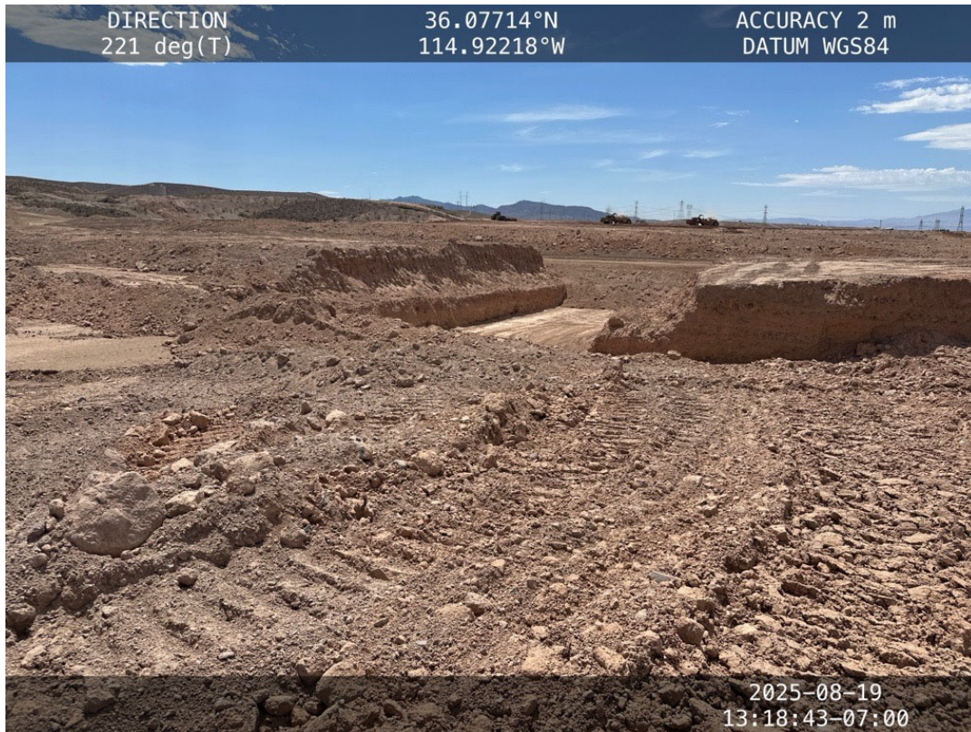
Cover Placement in Closure Unit 1 – August 19, 2025
