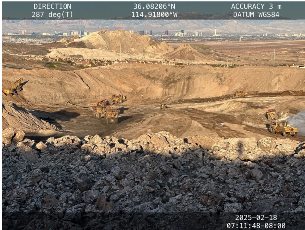
Waste Rock Reclamation in Tailings Pond 2 North – February 18, 2025
