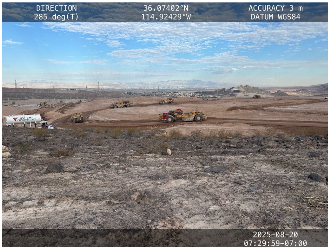
Cover Placement in Closure Unit 1 – August 20, 2025
