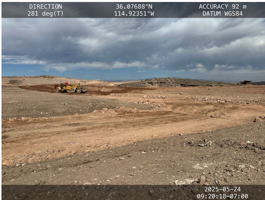
Cover Placement in Closure Unit 1 – May 24, 2025
