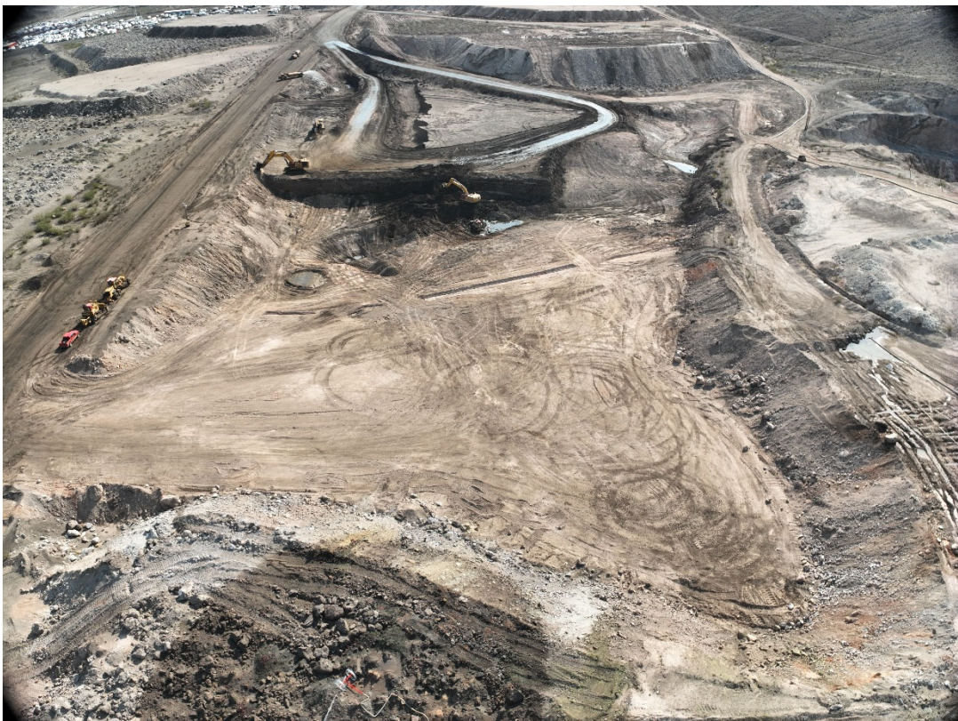
Tailings Pond 3 West – July 25, 2024
