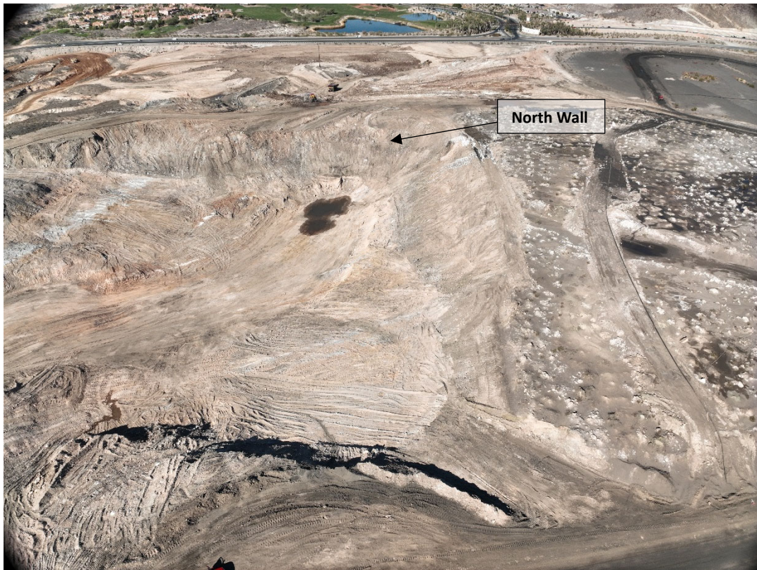
Tailings Pond 2 North – November 18, 2024
