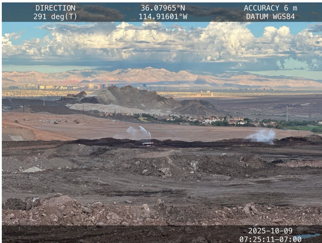
Pre-watering waste rock prior to movement in Closure Unit 1 – October 9, 2025
