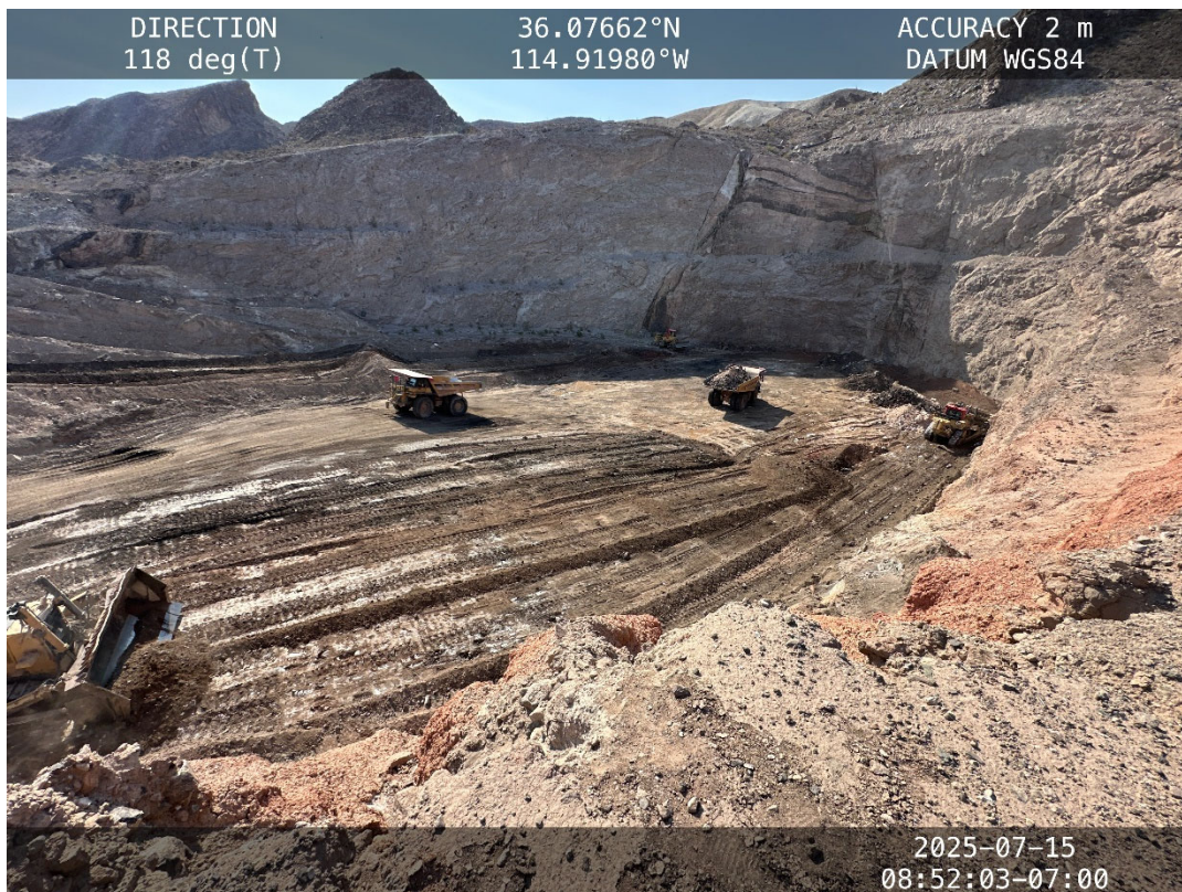
Waste Rock Reclamation in Closure Unit 2, backfill of the Hulin Pit – July 15, 2025
