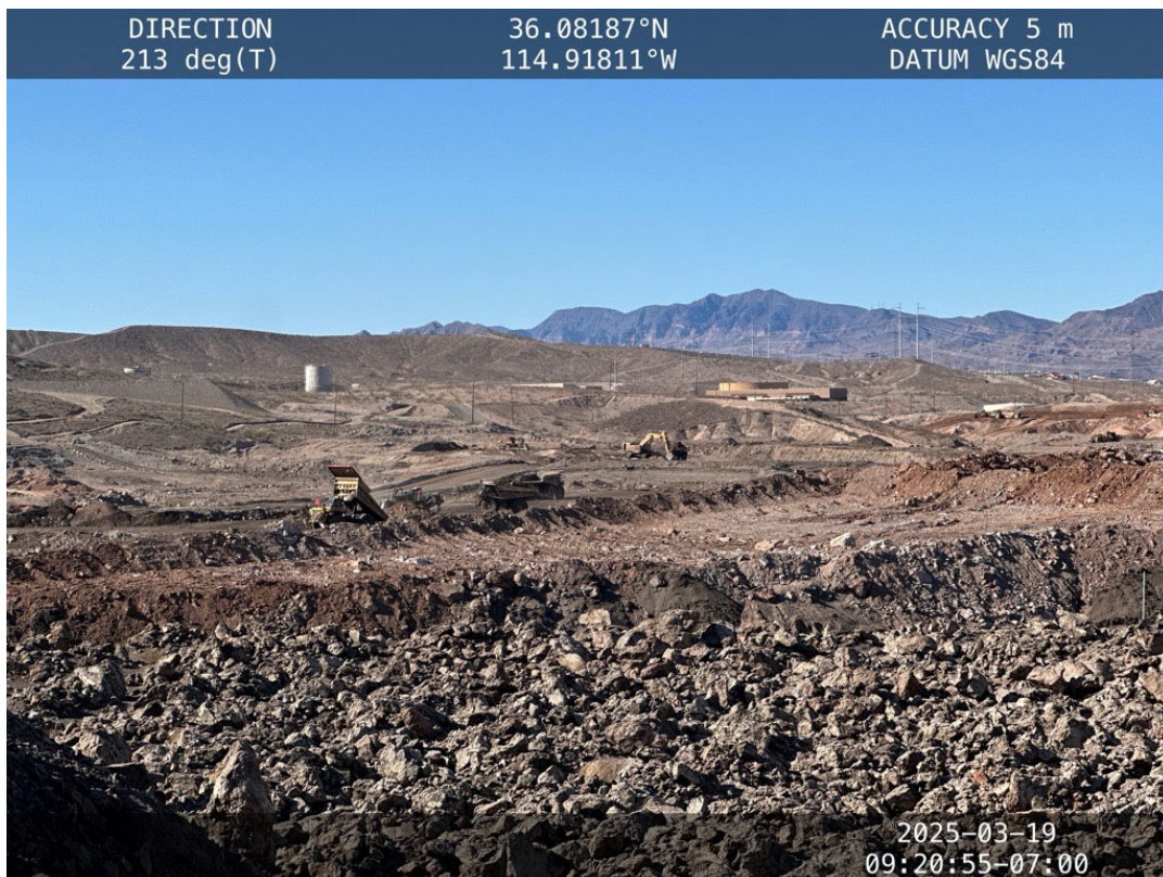
Waste Rock Reclamation in Closure Unit 1 – March 19, 2025
