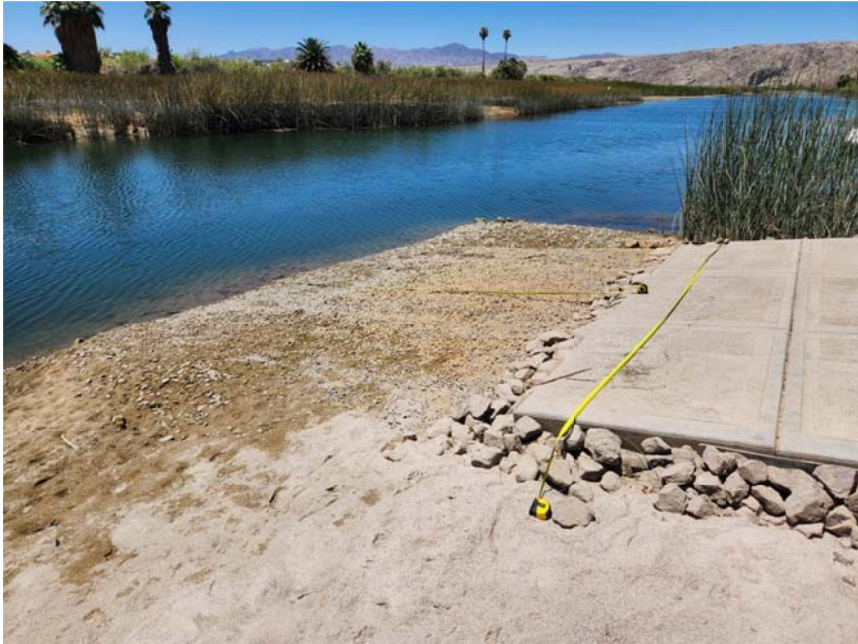
Photograph 6. End of existing boat ramp showing additional 16 foot extension request (8 feet concrete panel, 8 feet Enviro-Grid) with measuring tape; view facing west.
