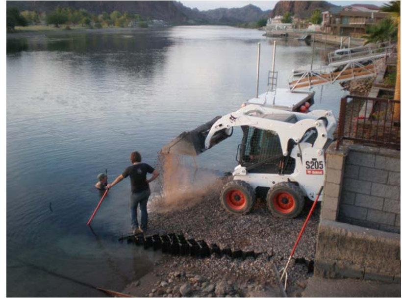
Filling Forms with Crushed Aggregate
