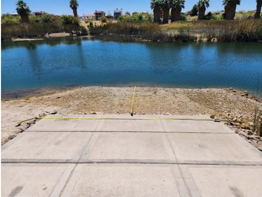
Photograph 5. End of existing boat ramp showing additional 16 foot extension request (8 feet concrete panel, 8 feet Enviro-Grid) with measuring tape; view facing south.
