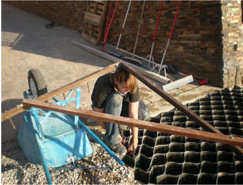
London Bridge Marine laying out GeoGrid Forms
